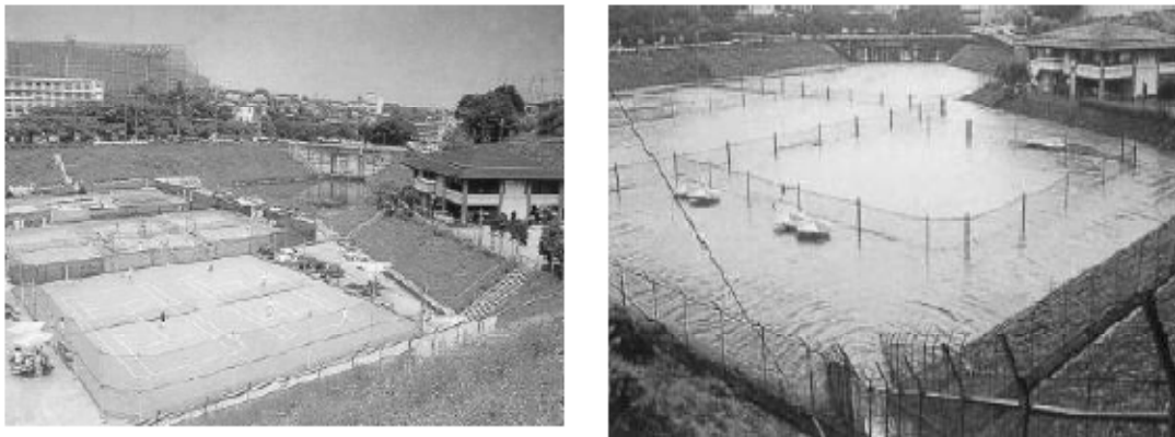
Figure 7-12: Example of Multipurpose Detention Basin in Japan (Associated Programme on Flood Management, 2008)
