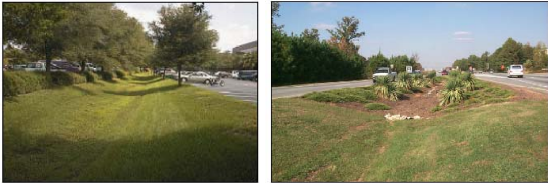
Figure 7-8: Profile View of Vegetated Swale (Portland Bureau of Environmental Services, 2004)
